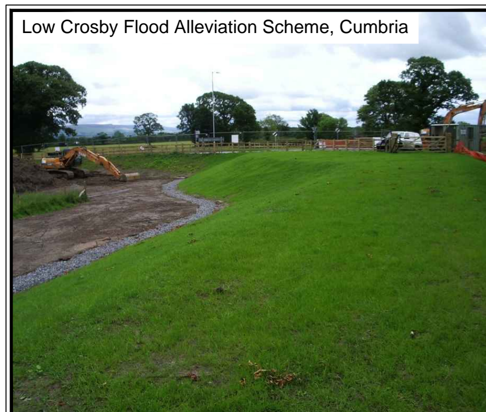
Flood defence embankment with grassed finish and gravel toe drain
