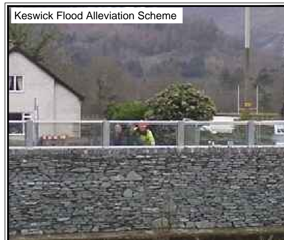
Natural stone finish with upper reinforced glass panels to improve flood protection whilst not severing the views of the river from the community
