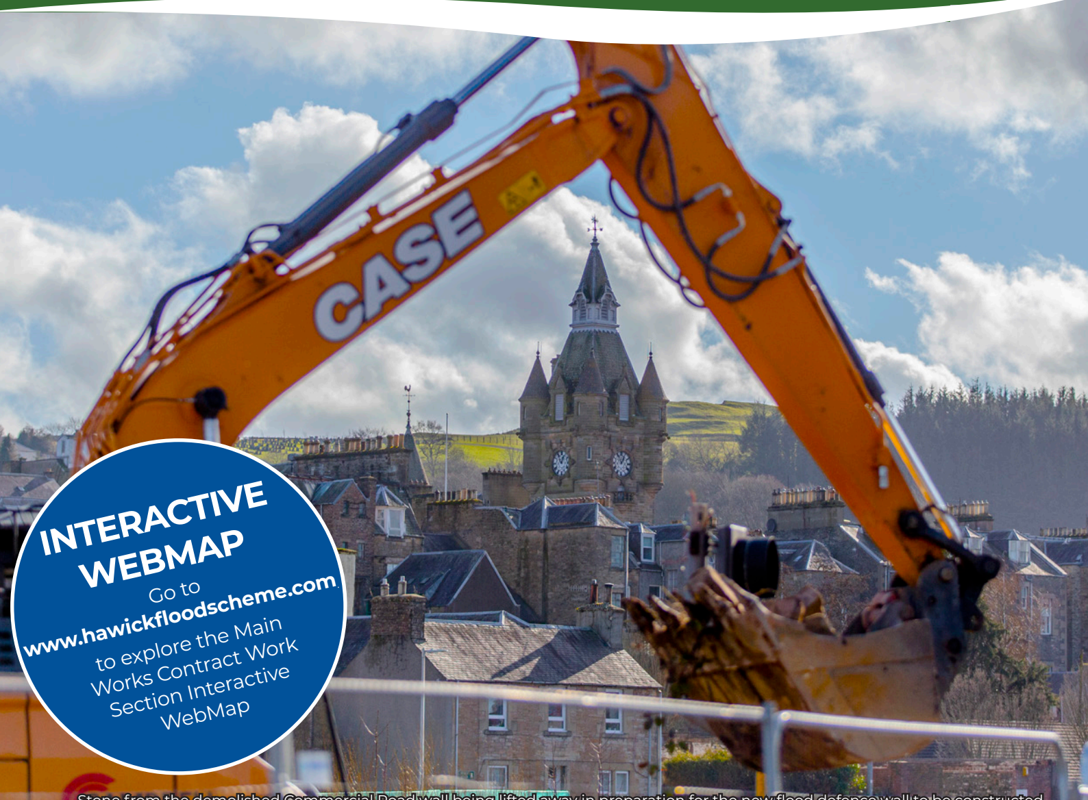
Stone from the demolished Commercial Road Wall being lifted away in preparation for the new flood defence wall to be constructed.
