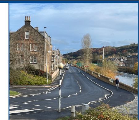
Mansfield Road reopen with two-way traffic and reinstated parking with traffic calming measures.
