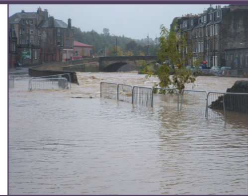
The river burst its banks and overtopped historic flood defences, causing major problems at Commercial Road in 2005.
