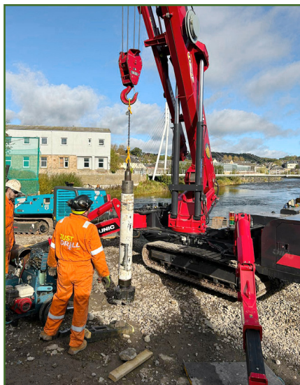
Specialist equipment to pile to required depths brought to site
