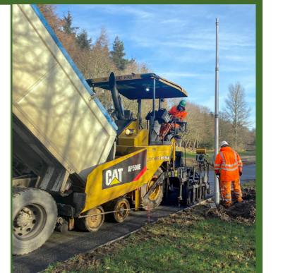
Tarmac surfacing works at Waverley Walk following streetlighting install.
