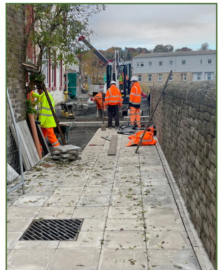
Footpath paving underway following the flood wall cladding finishing
