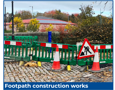
Footpath construction works
