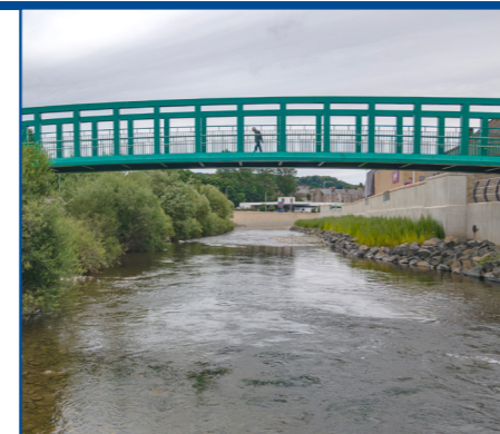
Victoria Footbridge was replaced with an elevated and wider 2.5 metre shared use crossing.
