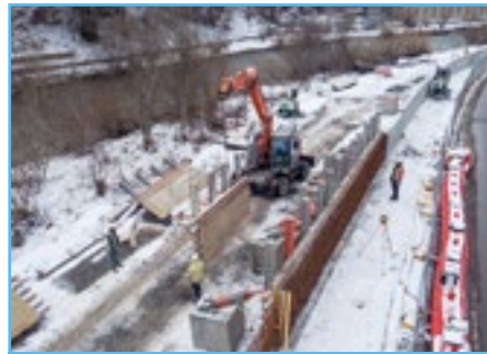
Shutters being lifted into place
