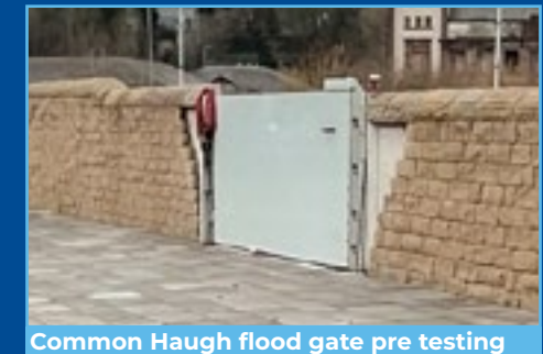
Common Haugh flood gate pre testing
