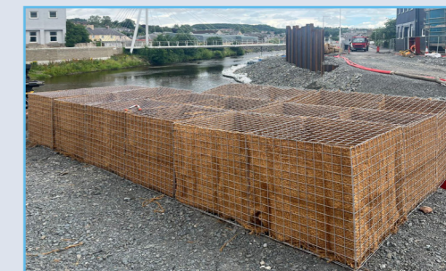
Straw bales on site before installation
