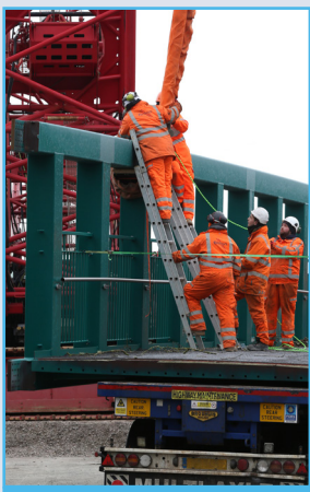
Footbridge lift safe site
