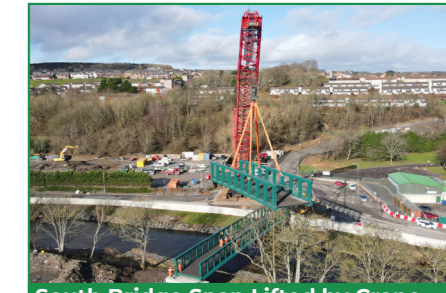
South Bridge Span Lifted by Crane
