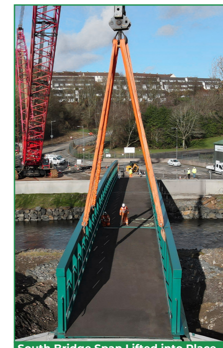
South Bridge Span Lifted into Place
